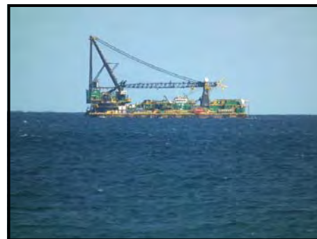
Barge putting down pipes for new rig
