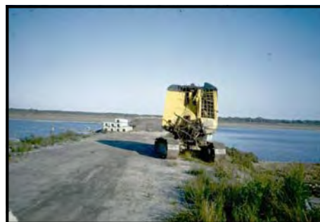
1st bridge under construction
